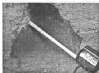
图5 无支护的空腔开挖图 Fig.5 Cavity excavation without support
